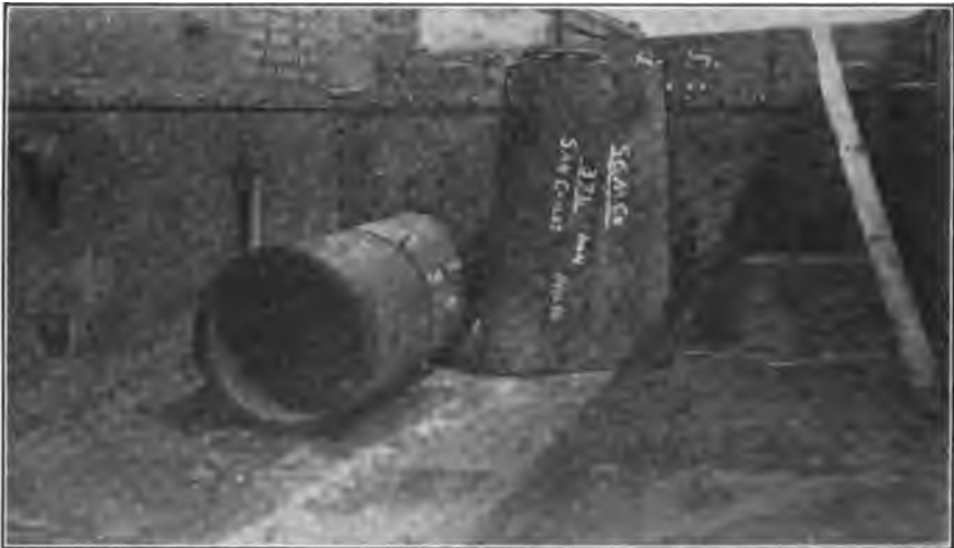
FIG. 147.—A 24-in. \times 40-ft. steel smoke-stack knocked down and nested for shipment. One bundle 30 in. \times 30 in. \times 57 in., 1,107 lb.; and one brichin 36 in. \times 36 in., 141 lb.
